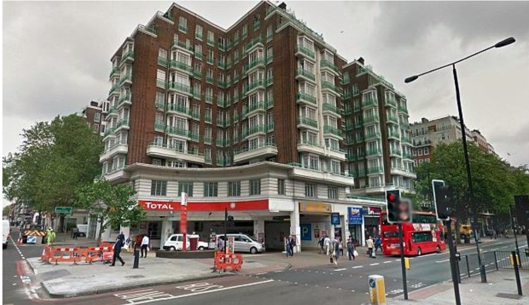
Dorset House, as seen from Marylebone Road with petrol station undergoing works (top) and prior to the fire in the underground car park (bottom).
